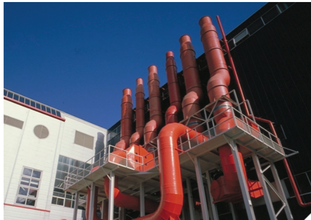
Industrial Facilities produce specifically toxic waste that is discharged to nodal treatment system
